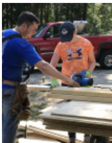
Matt Allen & Kelsey Phillips make a staircase for a homeowner.
